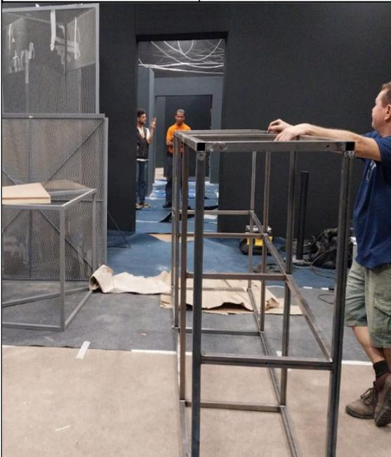
**FOTO 80:** Montagem auto portante da estrutura das salas expositivas. A photograph showing the installation of a self-supporting metal frame for an exhibition room. The frame is made of dark metal beams forming a grid-like structure. Large windows are visible in the background.
